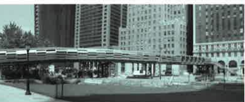
Rector Street Bridge under construction late June 2002. SHoP
