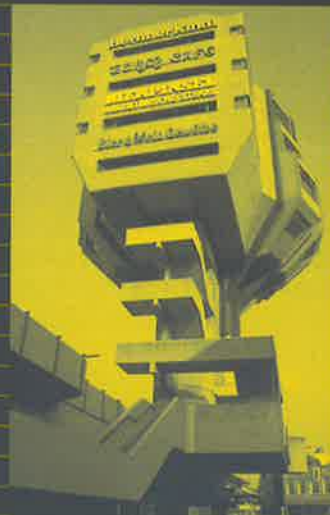
Structure on the Berlin Autobahnring. RALPH STERN
