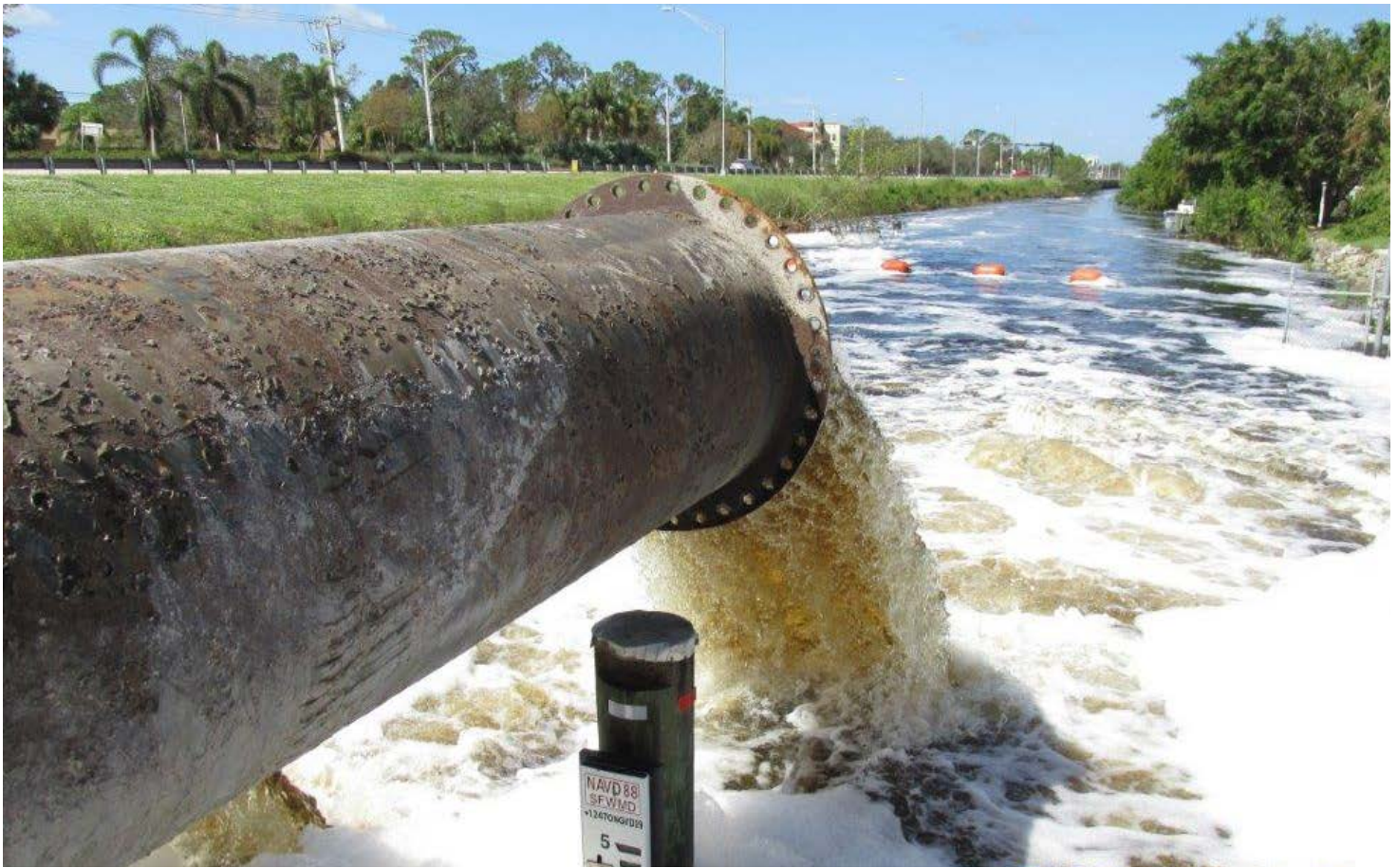
Fig. 2 Cocohatchee Weir 1 temporary pumps
