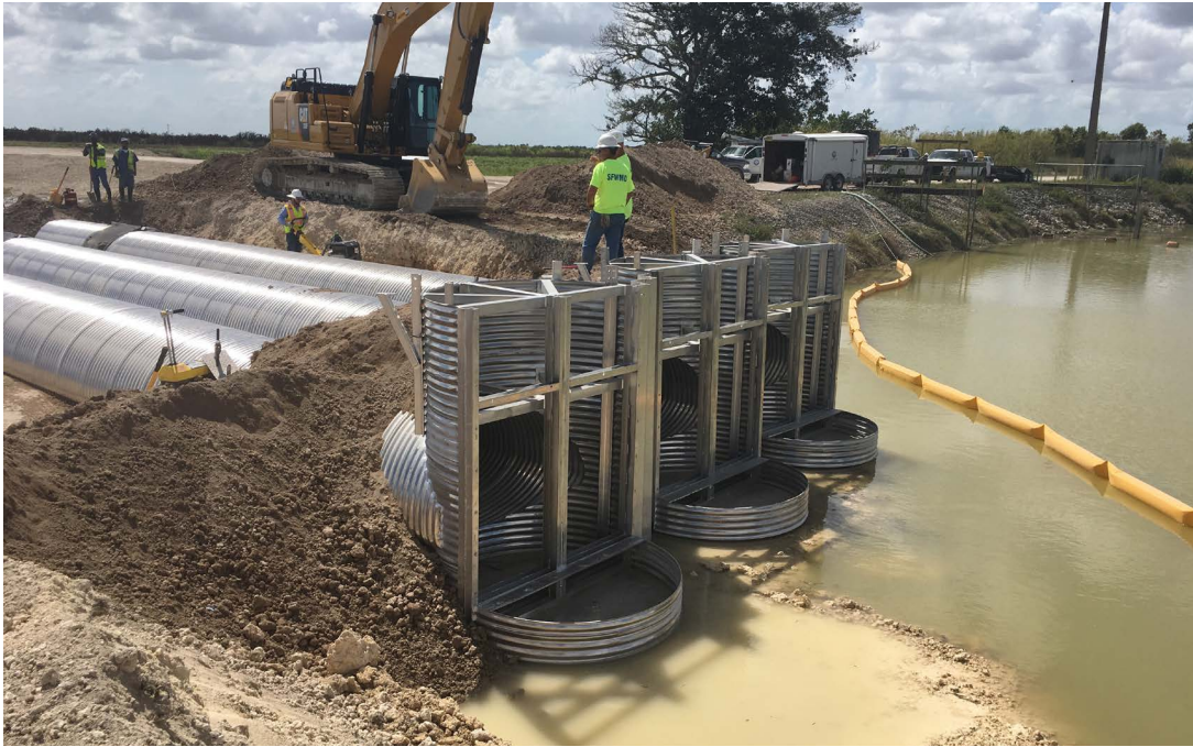
Fig. 1 Culvert installation
